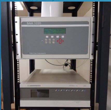
La Jolla's continuous PM 2.5 monitor and ozone analyzer in the rack.
